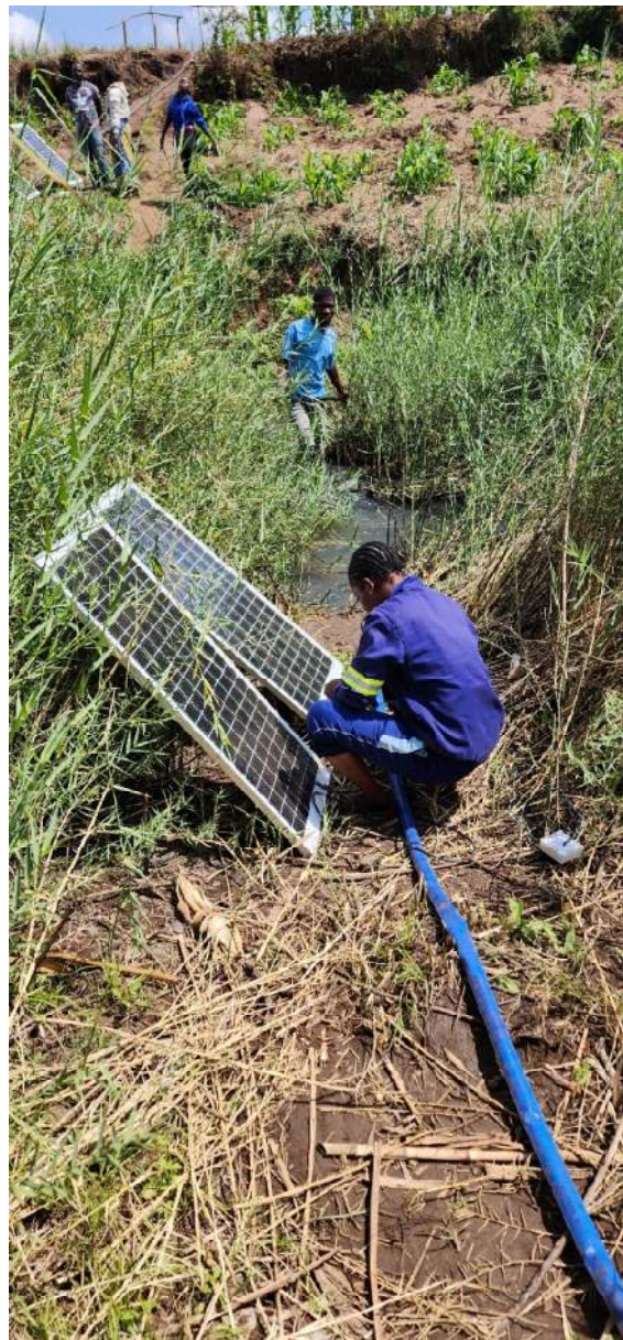
Figure 1: Typical solar irrigation pump system installed each day. Solar panels and Inflated lay-flat hose in the foreground, pump concealed in the stream beyond.
